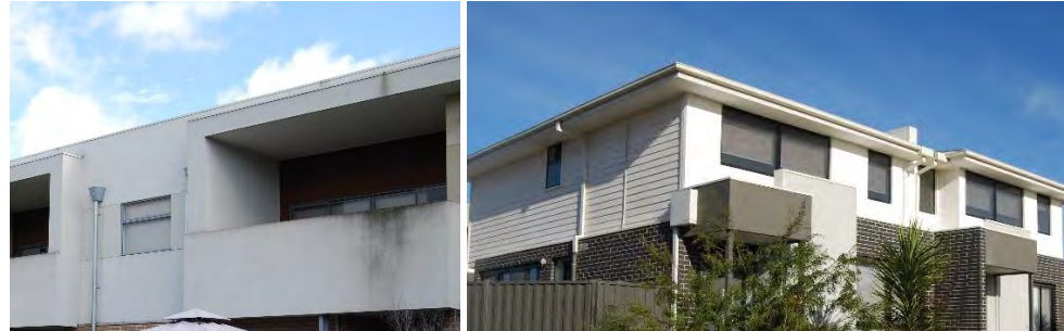
Figure 21: Example of poor-quality, water damaged material (left) and higher quality material (right)
