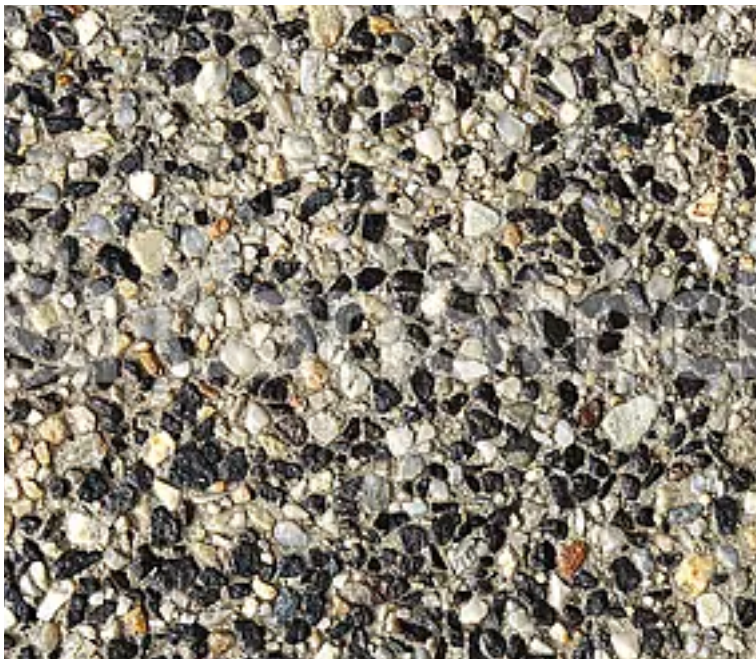
EXPOSED AGGREGATE CONCRETE PAVING
