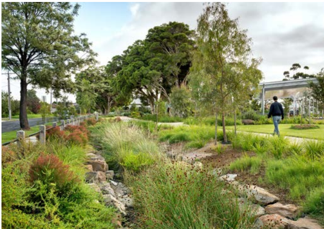
A vegetated swale WSUD asset as part of a storm water strategy
